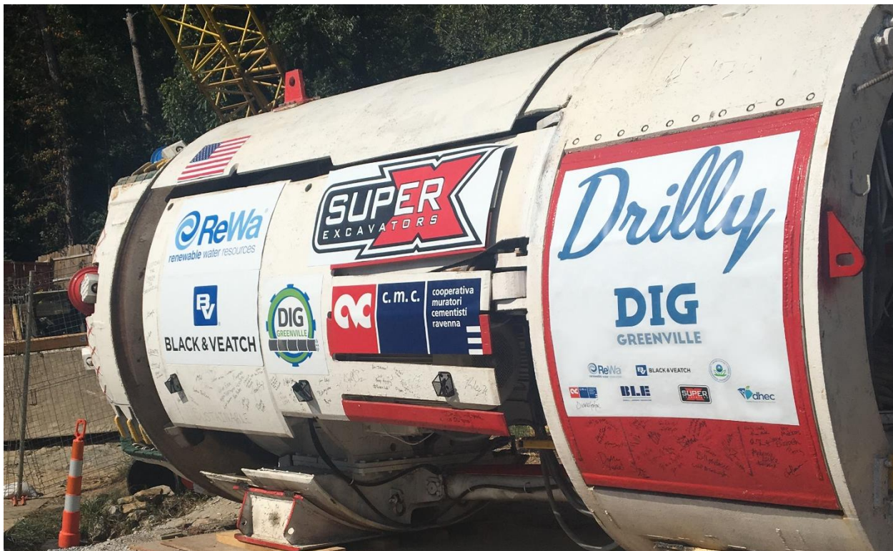
The Dig Project Tunnel Boring Machine
